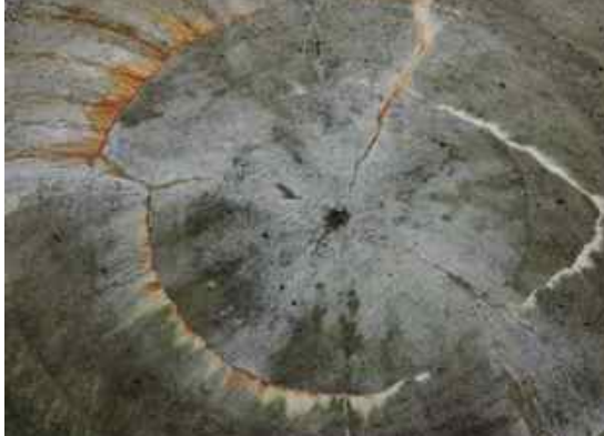
Concrete ceiling of Expansion Bell
