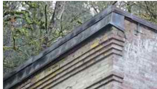
Front facade roofline
