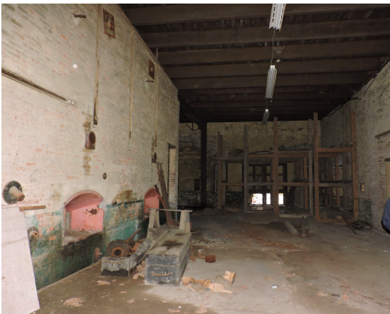
Central area, viewed from front entrance
