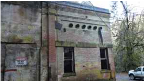
Rectangular double hung windows on front facade
