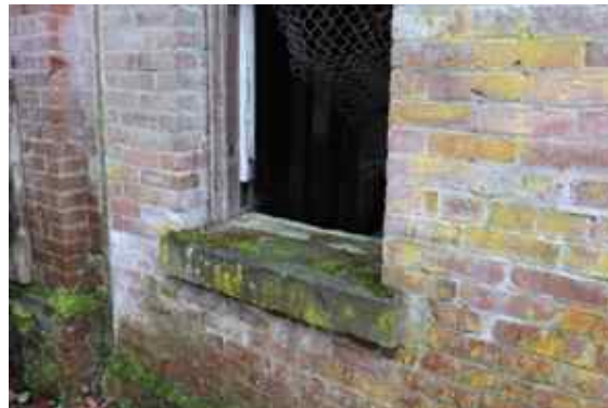
Front facade, window sill
