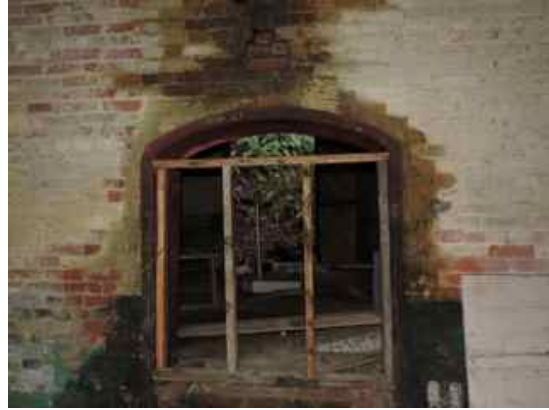
Opening to SW side addition
