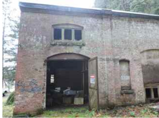
Rear facade; the door to the NE addition is open.
