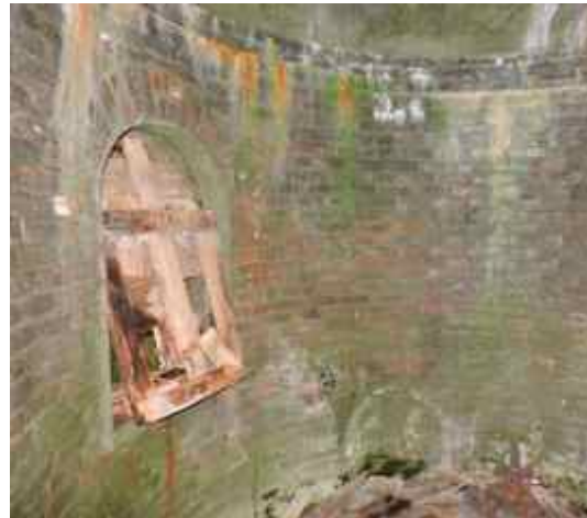
Interior of Bell structure, showing brick construction and damaged window screen
