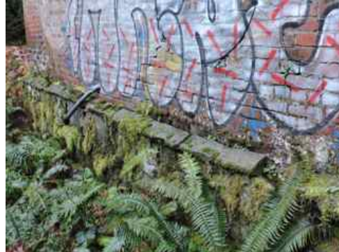
NE facade, foundation
