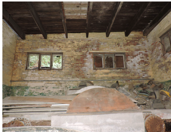
Alcove on the left at the back of the central area, used for storage
