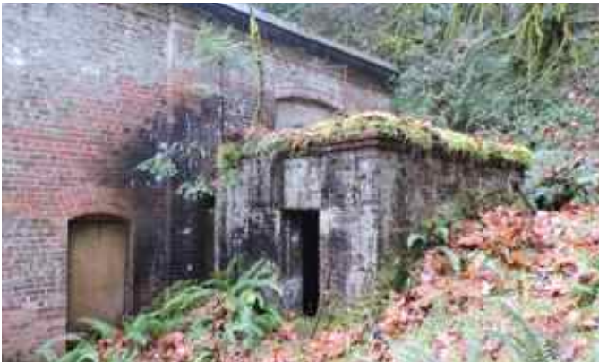
Exterior bunker, south side of Powerhouse
