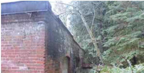
SW facade roofline
