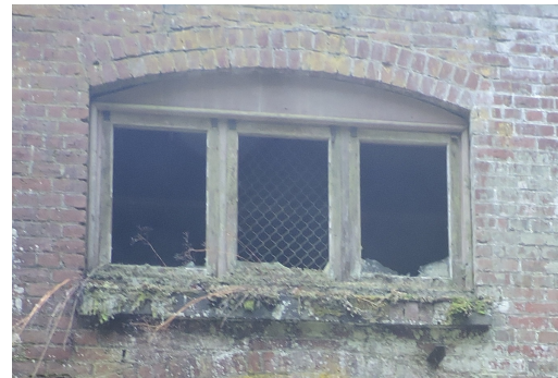
Rear facade, relatively intact window
