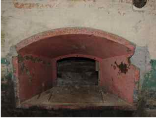
One of two Pelton Water Works (dated 1898) throughways to SW side addition – may allow the shaft of the water wheel to connect with generator
