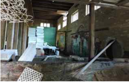
Water trough (?) and sealed round openings on exterior (NE) wall, viewed through window on north facade.
