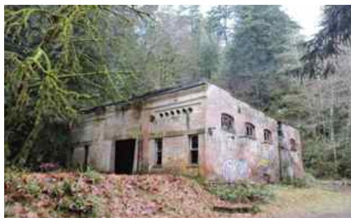
Goldstream Powerhouse in 2016, front and NE facades
