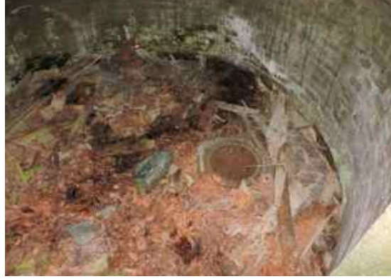
Floor of Expansion Bell, showing pipe opening
