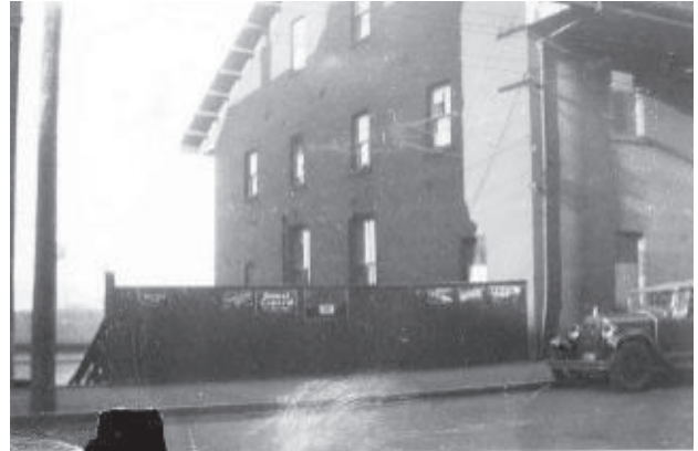
PHOTO 15: likely taken at the same time as Photo 13, the pedestrian access stair can clearly be seen to the left.
