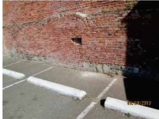
PHOTO 17: South elevation 1930's
