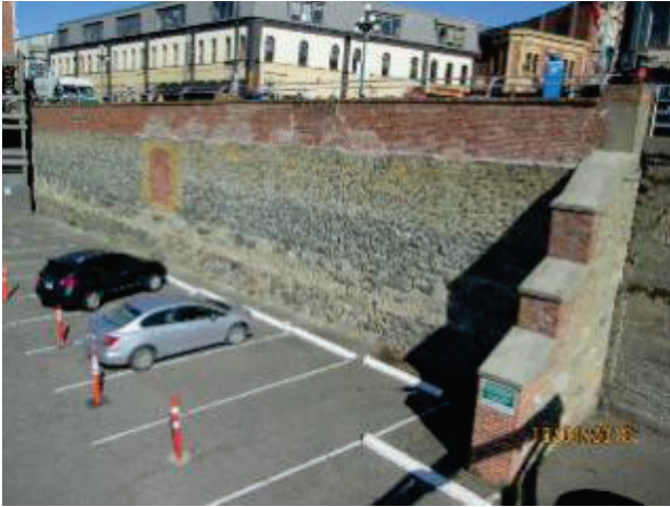
PHOTO 2: SECTION 1 , formerly part of the Hudson's Bay Company Warehouse.
