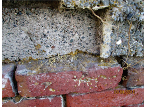
PHOTO 48: Closeup of the cast in place concrete door sill complete with an outline and profile of the wooden door frame and mouldings.
