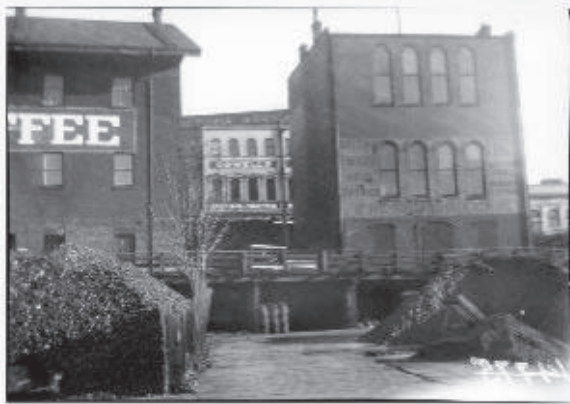
PHOTO 14: Showing the timber platform between the two warehouses.
