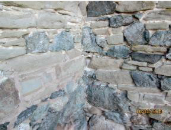
PHOTO 41: Close up of the inside corner of the buttress.
