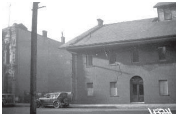
PHOTO 13: Wharf street looking west showing the gap between the two buildings
