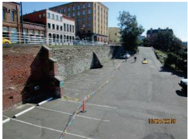
PHOTO 5: SECTION 4 , Stone retaining wall.
