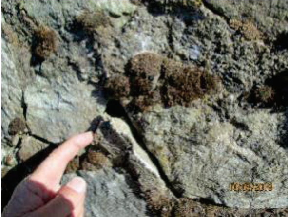
PHOTO 80: Failed mortar joints, cracks vary in width from 10mm to 25mm.
