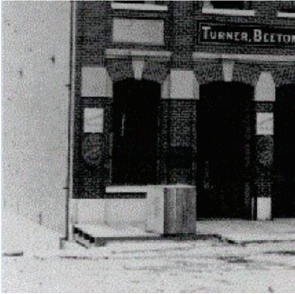
PHOTO 24: Enlarged view of the Turner Beeton Building. In the foreground the sidewalk appears to be suspended between the building and the line of the stone retaining wall.
