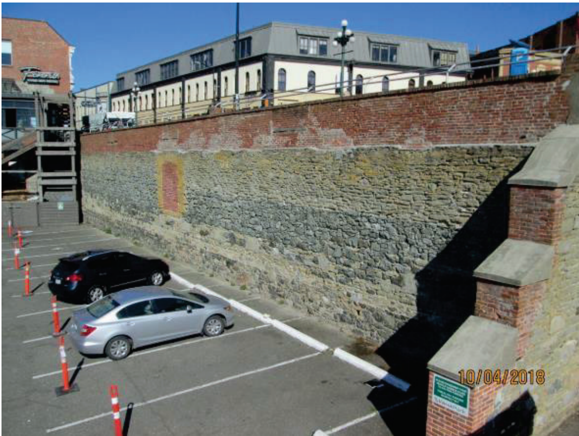
PHOTO 30: A general view of SECTION 1 showing the different construction materials.
