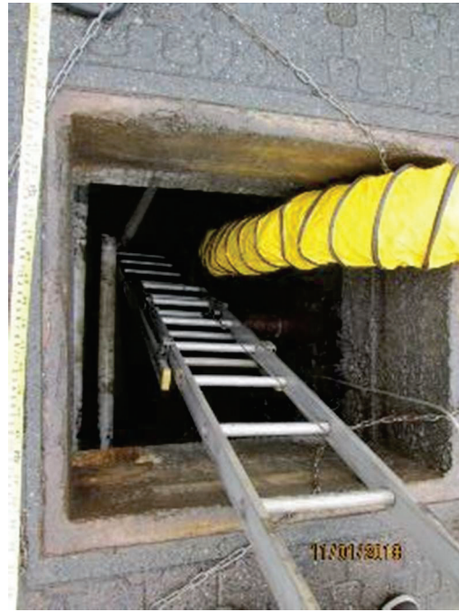
PHOTO 52: Access was gained using confined space protocols.
