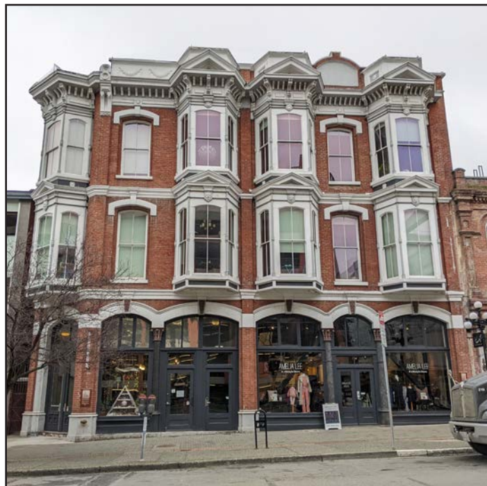
Figs. 3.1a & b: Example late 19th and early 20th century brick buildings in British Columbia. The bottom building has had some retrofit work done, as visible in the store window with the black diagonal bracing. (Sources: Katie Cummer)
