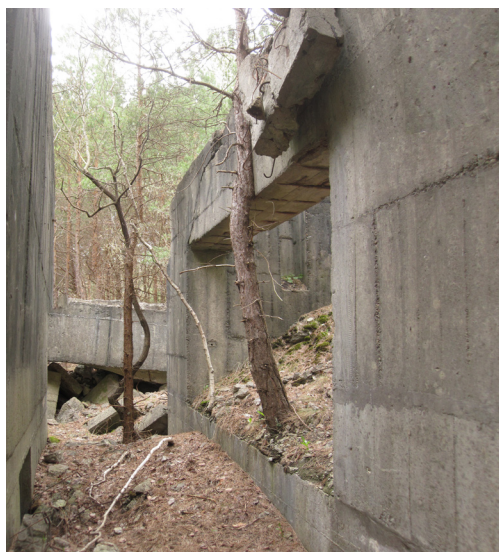
Fig. 5: Actual state of ruin – left side (a): concrete 'bloc C', remaining part of the basement of F1. Spring 2016. Possible lift shaft (photo merge: P. Schneider); right side (b): pre-cast concrete elements in eastern part of 'Rampe' area (photos: P. Schneider).
