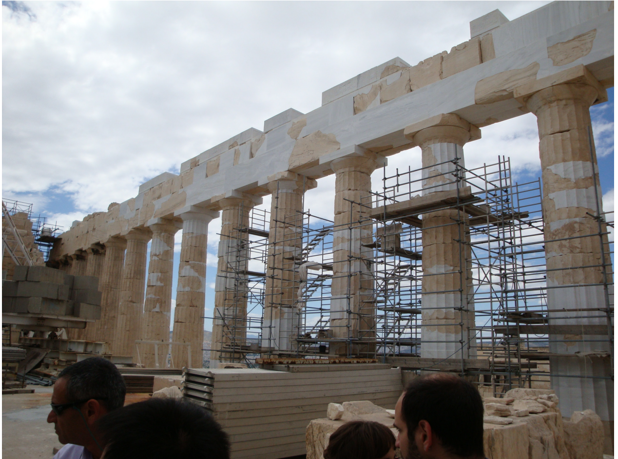
Fig. 7: The anastylosis restoration of Parthenon, Athens. The Venice Charter states that all reconstruction work should be ruled out 'a priori' and only anastylosis is permitted (Photo: Bijan Rouhani).
